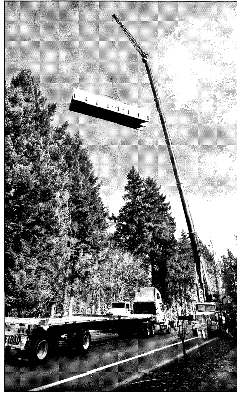
(left) A Campbell Crane lifts a 15,000-pound wooden bridge 180 feet in the air and 210 horizontally...
